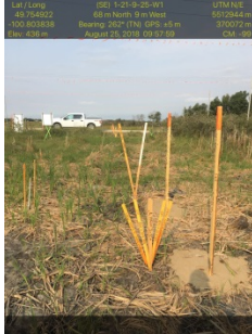
Aug 25/18 SSKP 821+112 Wetland Complex Class 5 Facing West towards gravel road Stakes indicating bore and buried lines With overhead powerline safety rope above
